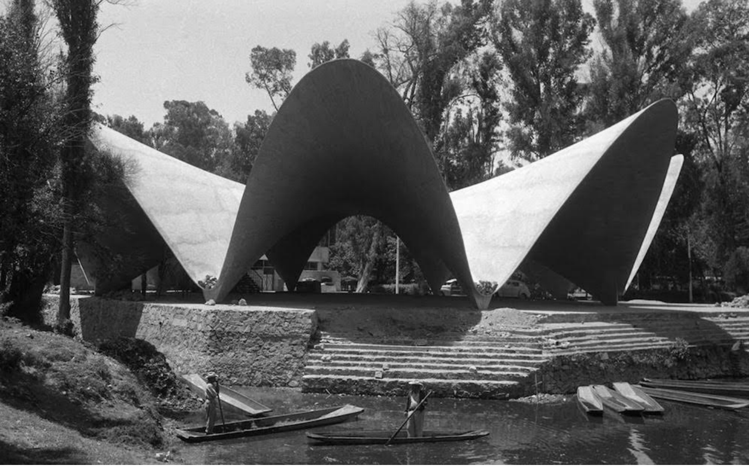
Los Manantiales Restaurant, Mexico City
