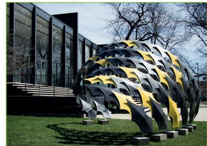
Carbon Fiber structure called ‘FIBERwave Pavilion’ designed by IIT Architecture students led by Alphonso Peluso 2014
